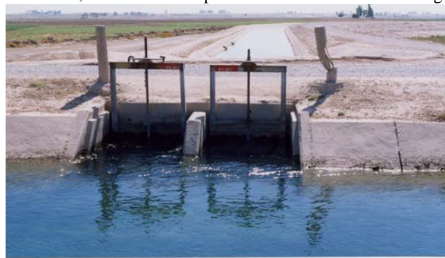
Fig. 3 A cross-regulator in a main canal
