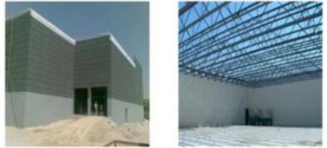
Fig. 12: Dafza project, Royal City Contracting LLC[17]
