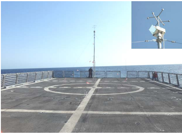
Fig. 6 Sonic anemometer installed in the flight deck
