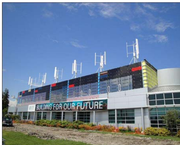
Fig. 4 Example of VAWT installation on the roof of an urban building (from: [20])
