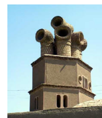
Fig. 6 Pipe Shape Wind-catchers
