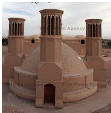
Fig. 1 Dolatabad Wind-catcher, Yazd
