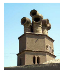
Fig. 6 Pipe Shape Wind-catchers
