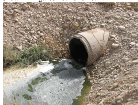
Fig. 1. Effluent of yasuj waste water treatment plant
