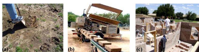
Fig. 20 Soil as construction material. (a) soil on Hudson Farm, (b) CEB machine making blocks; (c) a house under construction using CEB in New Mexico
