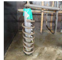
Fig. 5 Shape of the Spiral Bar
