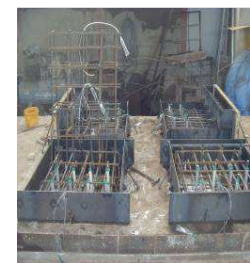
2. Installing Cast and Placing on Concrete Deck
