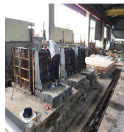
3. Installing Cast and Placing Concrete in Barrier
