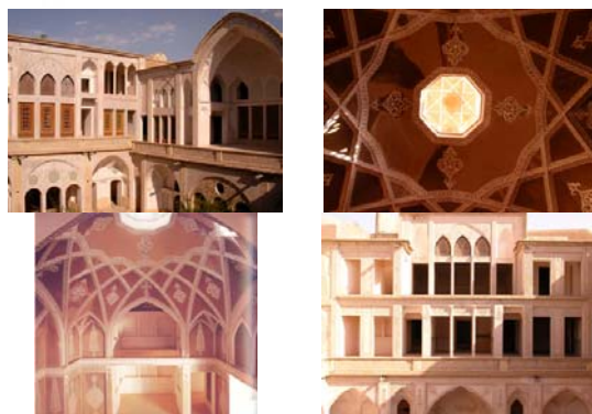
Fig. 4 several views of Abbāsid house in Kashan
