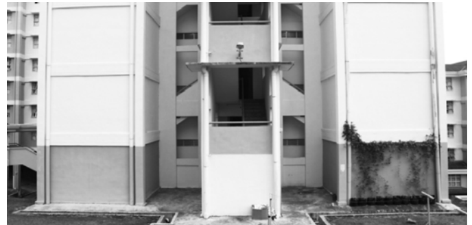
Fig. 5 Typical room (exposed wall) on the left and biofacade room (plant shaded wall) on the right. The walls were painted with light peach. The picture was taken when P. tetragonobulus at 3-4 months old.
