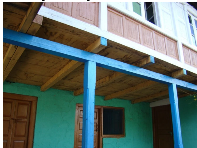
Fig. 6 Timber flooring and cantilevered balcony
