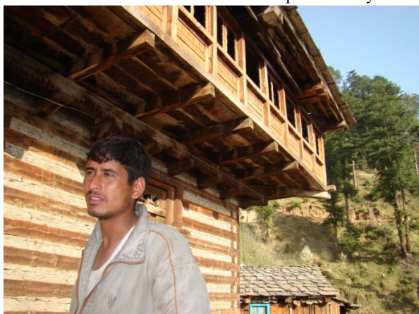
Fig. 5 Traditional 'Kath-khuni' wall construction with timber & stone
