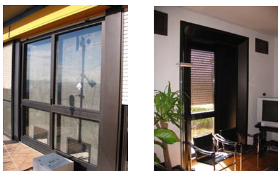
Fig. 1 Outside and inside view of solar wall
