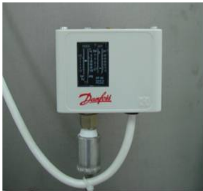
Fig. 10 Pressure sensor
