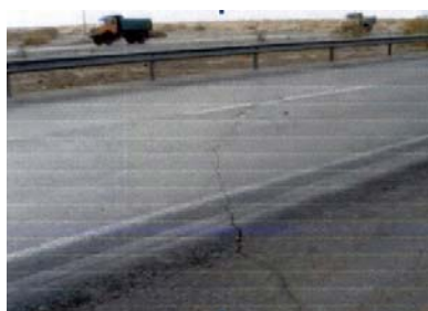
Fig. 5. Fissuring in Yazd-Maybod main road
