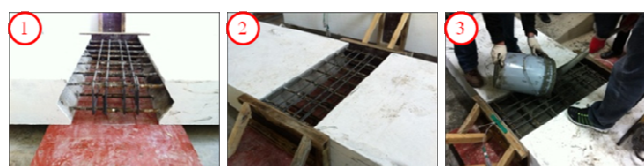
(a) Precast members (b) Setup the mold (c) Placing concrete
