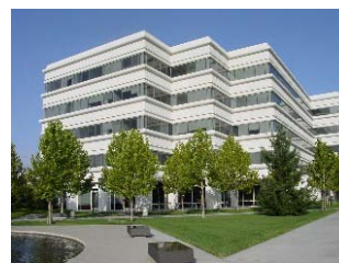
Fig. 1 The building of the Bishop-Ranch
