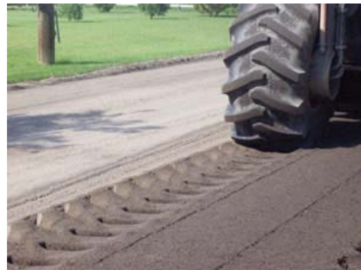
Fig. 2 Blending fly ash with pulverized base material
