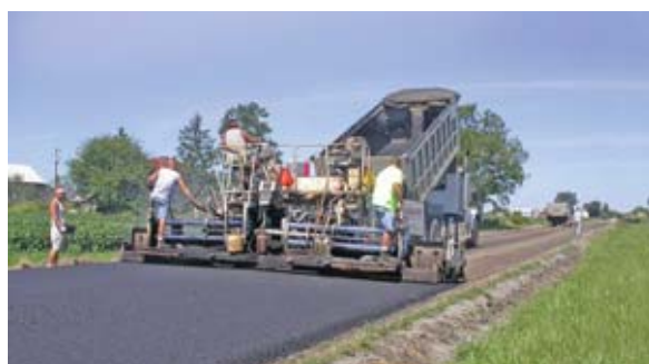
Fig.4 Resurfacing with hot mix asphalt
