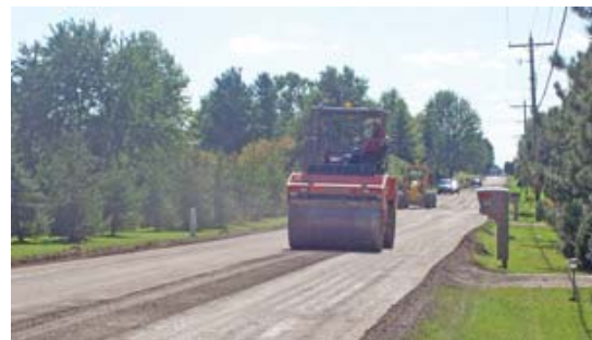
Fig. 3 Compaction of FDR base layer
