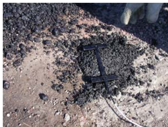
Fig. 6 Placement of strain gauge at top of FDR layer
