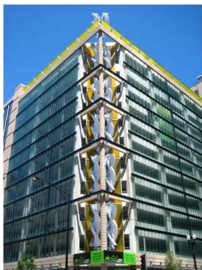
Fig. 2: Greenway Garage, Chicago (Illinois) (from: [7] [8])
