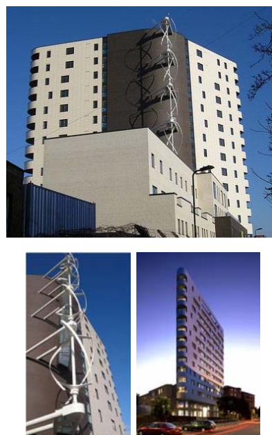
Fig. 6: Kinetica Building in Ramsgate Street [21], London (United Kingdom)
