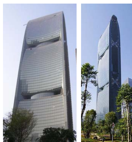
Fig. 4: a-b) Strata Tower [15], London (United Kingdom); c-d) Pearl River Tower [16], Guangzhou (China).
