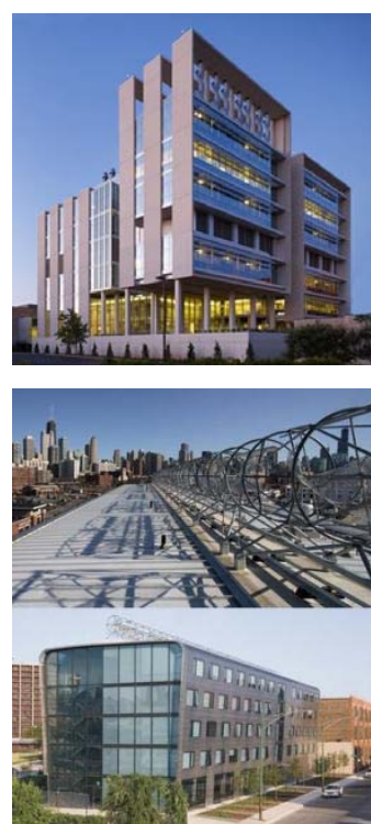
Fig. 7: a) Oklahoma Medical Research Foundation Building, (Oklahoma); b-c) Mercy Lakefront SRO, Chicago (Illinois).
