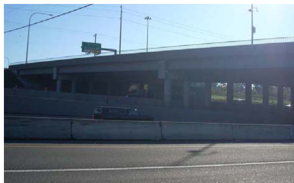
Fig. 2: Photograph of the Bridge
