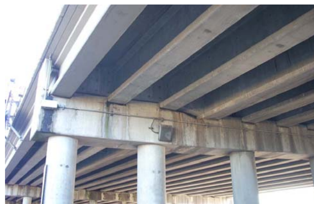
Fig. 3: Photograph of the Precast Girders at Pier 3
