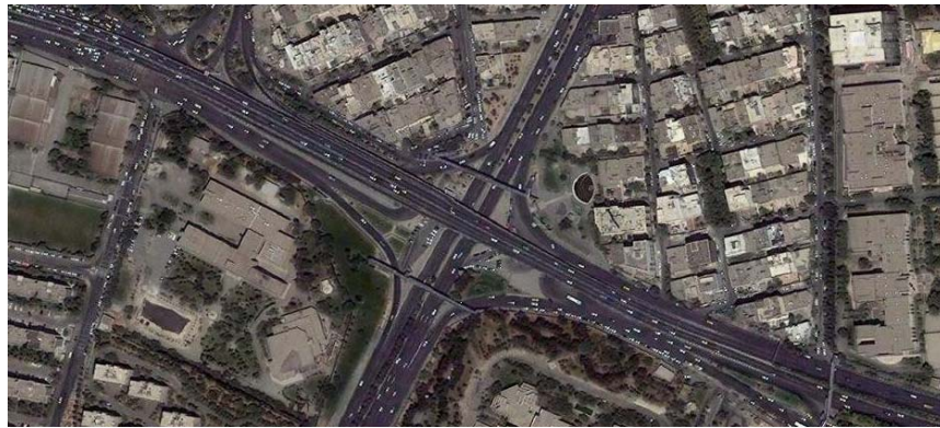
Fig. 2 Aerial Photo from Gisha bridge in Tehran City
