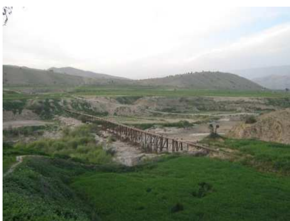
Fig. 6 The oil pipe line is located on the upstream of Kowsadam basin next to Choram , station 4
