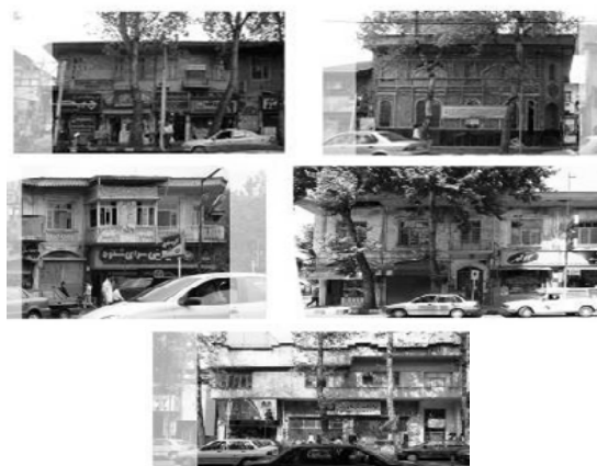
Fig. 3 Historical building facades with highest mean
