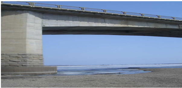
Fig. 1 (b) T-shape cantilever structure
