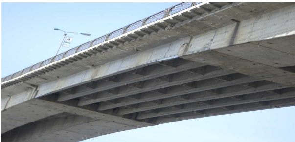
Fig. 1 (c) Hanging beams
