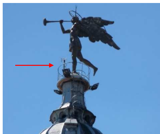
Fig. 3 View of the weather vane on the top of the bell tower of Lendinara; the red arrow evidences the location of the anemometer
