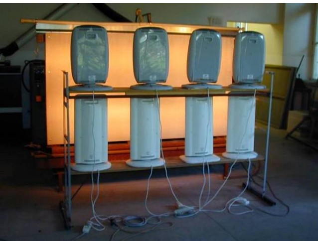
Fig. 16 Warming fiber-cement slab: view to electric warm sources
