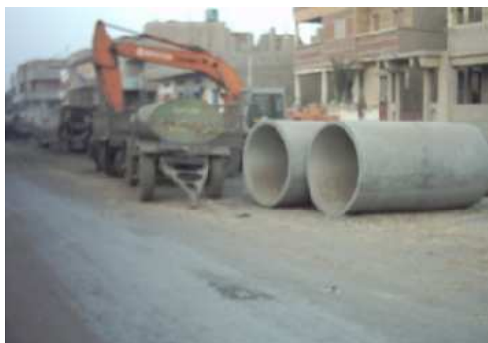
Fig. 3 Differential settlements in the pavement of the studied area
