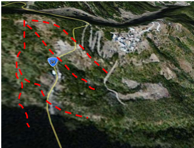
Fig. 13 Collapse Zone of Linear Structure (Google Earth)
