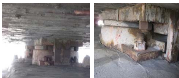
Fig. 8 Bearing steel plate
