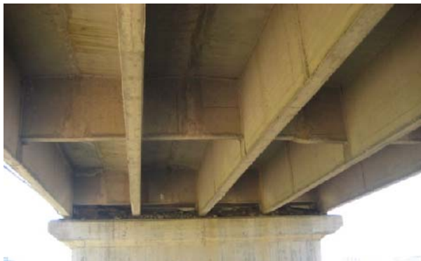
Fig. 9 (d) T Beam connections is good, no obvious damage (diaphragm)
