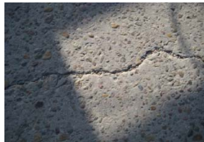
Fig. 10 Deck Damage
