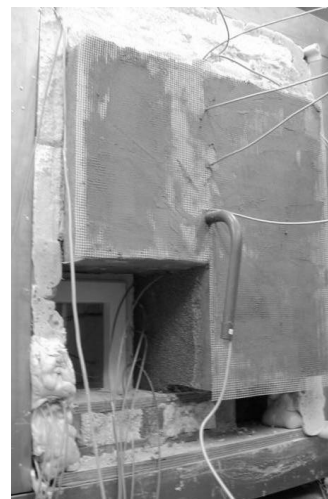
Fig. 4 Application of the insulation layer
