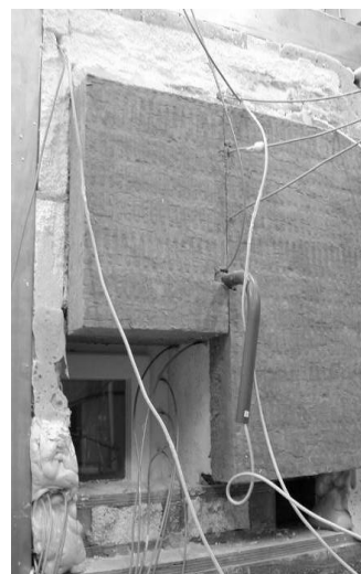
Fig. 5 Plastic net for plaster application
