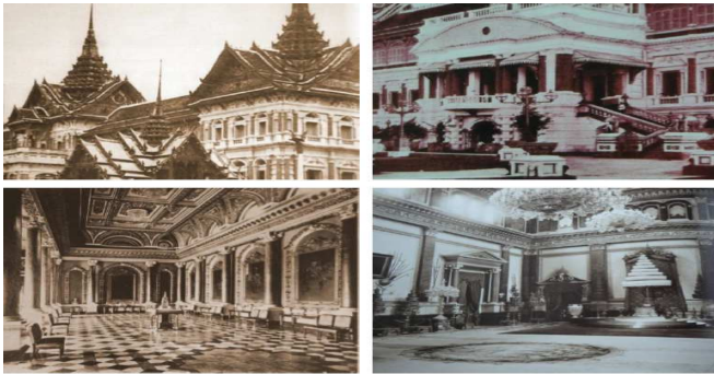
Fig. 14 Decoration Arts Before restoration of Chakri Maha Prasart Source: P. Povatong, Architecture in the reign of King Chulalongkorn , Bangkok: Amarin Printing & Publishing, 2010
