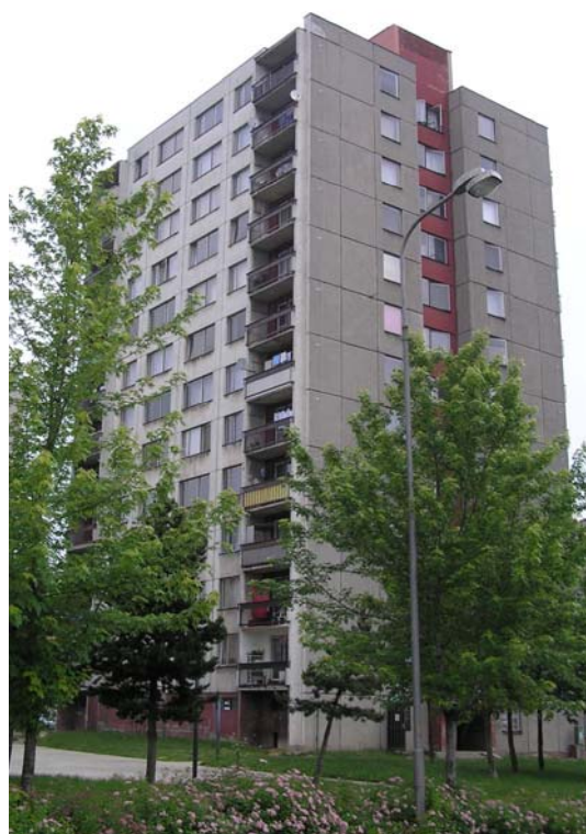
Fig. 1 Selected twelve storey residential building
