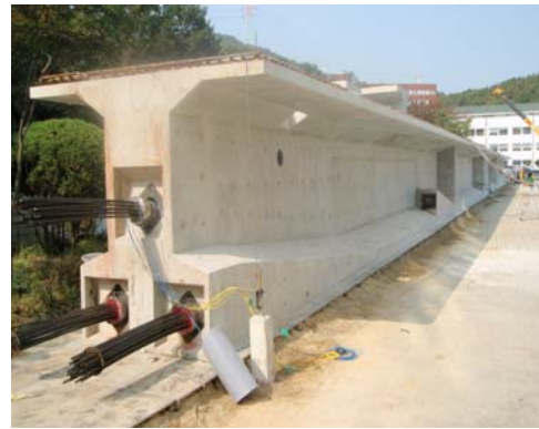
Fig. 12 Field test of anchor head load cell
