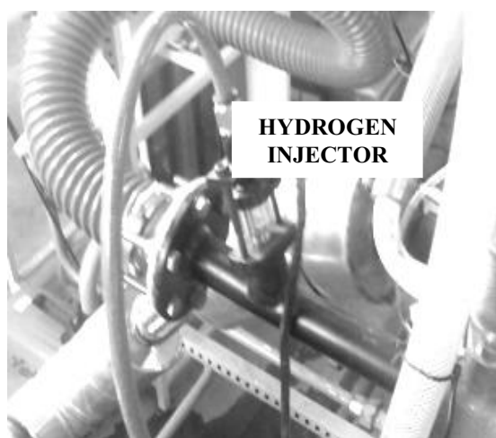
Fig. 2 Photographic view of the manifold injector
