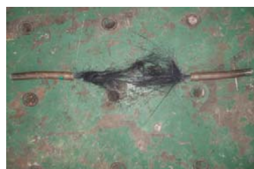
Fig. 11 Failure pattern of 7-multi CFRP tendon
