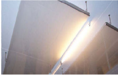
Fig. 23 Resonator placed on the ceiling
