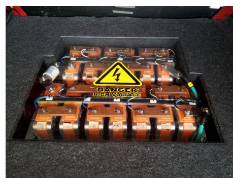
Fig. 4 Battery module arrangement within the EV boot
