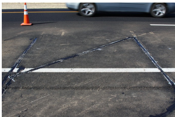
Fig. 5 Installation of axle sensing strips
