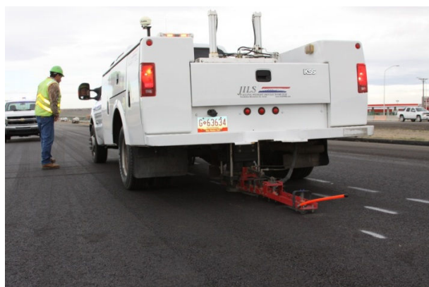
Fig. 7 Conducting FWD test
