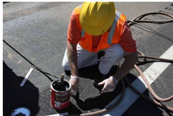
Fig. 6 Installation of temperature probes
