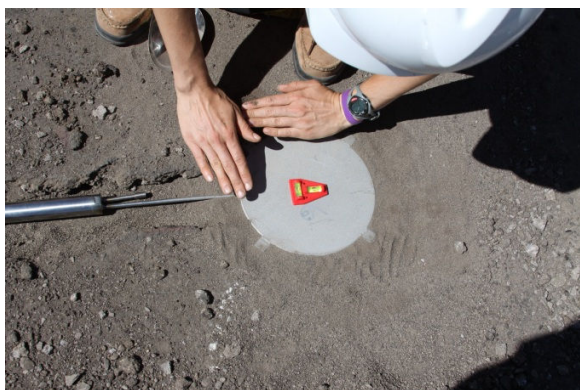
Fig. 4 Installation of earth pressure cell
