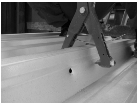
Fig. 6 Punch plies and hole for position threaded bar
