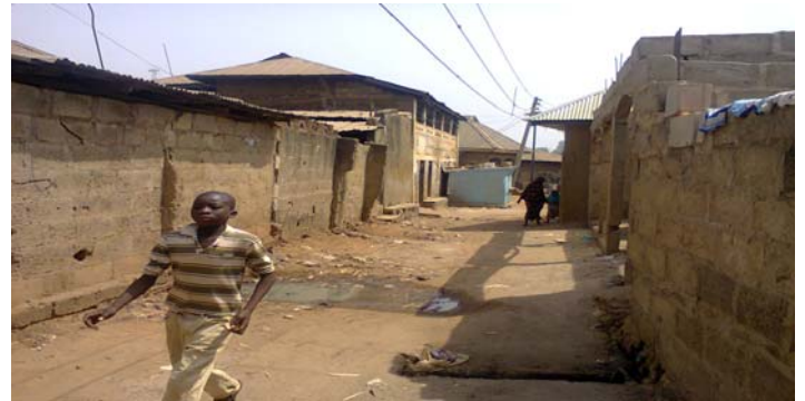
Fig. 4 Dilapidated structures in Zone C (Ungwar Doka)
