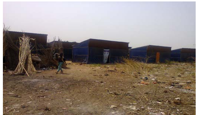
Fig. 3 Shanting structures in Part of Zone D
