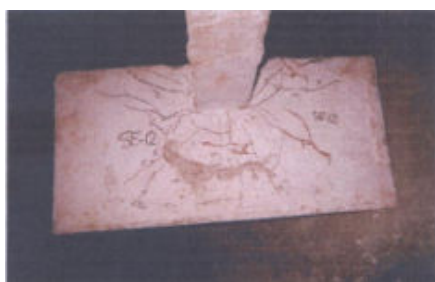
Fig. 2 Crack pattern as exhibited by Se-12
