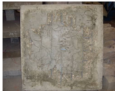
Fig. 19 Shape of cracks at bottom face for S1 Exp. (crack mode)
