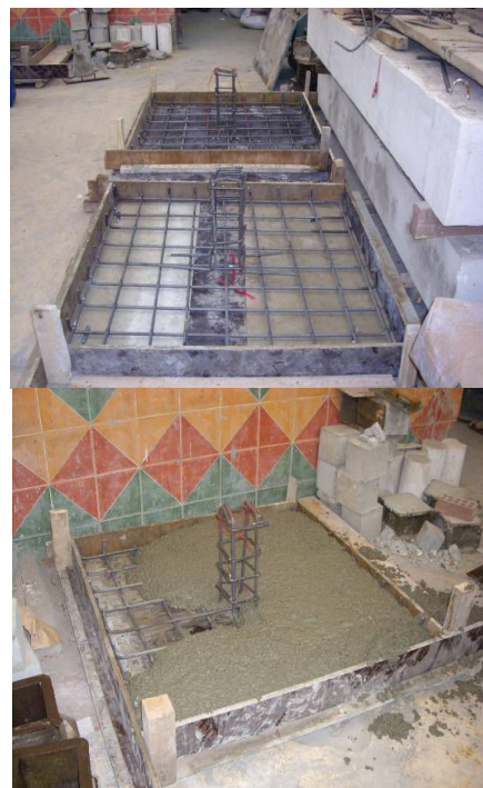
Fig. 1 Details of steel reinforcement and self compacting concrete
