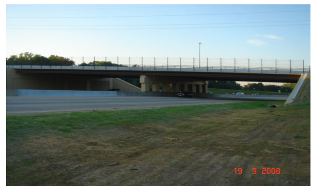
Fig. 1 Pacific Street and Interstate 680 Bridge, Omaha, Nebraska
