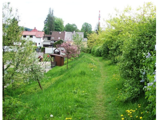
Fig. 4 Crest of extinct pond dam and urbanization in former pond area on the left side (pond ID 10)
