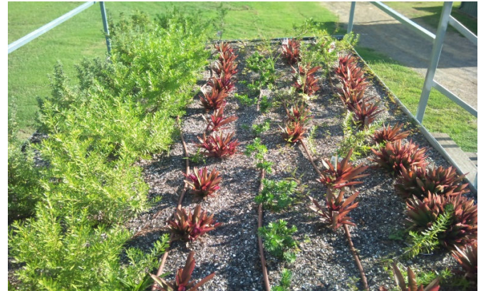
Fig. 3 Extensive green roof plants
