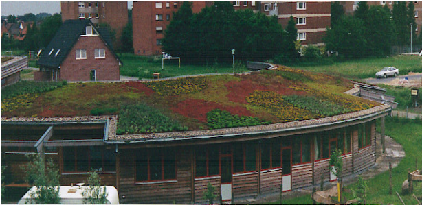
Fig. 2 Green roof at office/ school complex in Germany [10]
