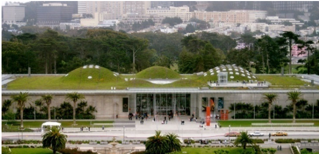
Fig. 3 Green roof on California Academy of Sciences [11]
