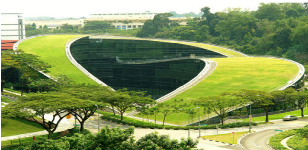
Fig. 4 Green roof on school of Art, Design and Media at Nanyang Technological University in Singapore
