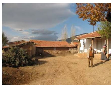
Fig. 3 Addition to the post-disaster house and new buildings on the lot (Kızıllı Village)
