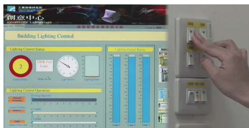
Fig. 9 Selecting of the lighting mode by using regular light switch
