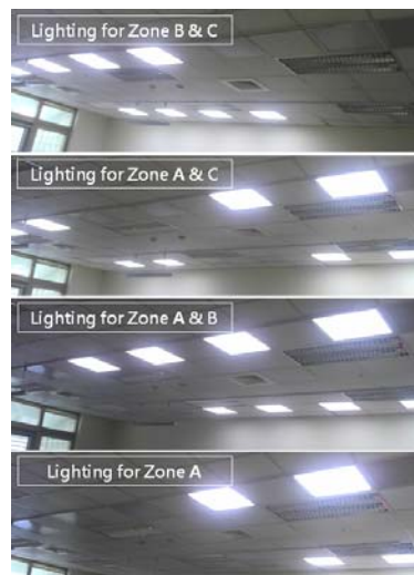
Fig. 11 Controls for dedicated lighting zone
