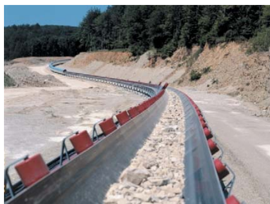
Fig. 1 Conveying limestone material on curved belt conveyors [12]
